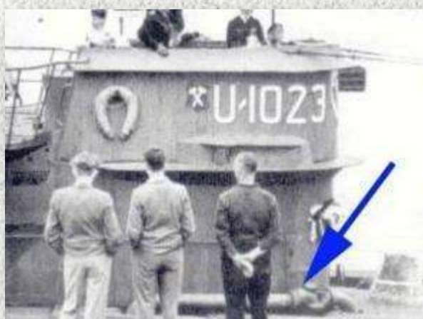
Left (C39): When the schnorchel was fitted a pipe was added on the deck, just to the port side of the tower. The blue arrow points to the pipe.
